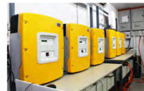
The Fuzzy controlled energy storage system that consists of bi-directional inverters, namely Sunny Island 5048 integrated with valved-regulated lead acid (VRLA)
