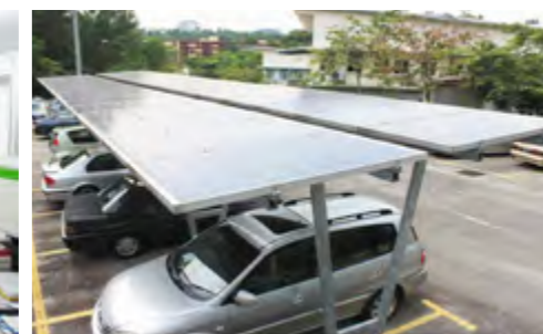
Photo-voltaic (PV) panels mounted on a 3.3 metre structure at the car park, K L campus
