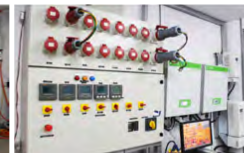
From left: the low voltage panel, two units of 3.6 KWP single-phase Photovoltaic inverters (middle) and the two variable speed drives
