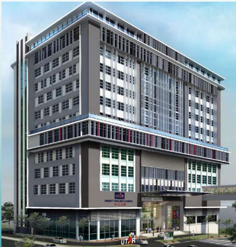
The new city campus building is expected to be ready by 2014.
