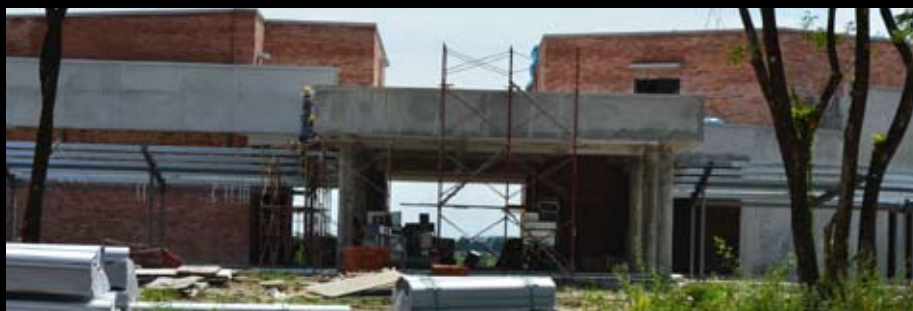
Lecture Complex II (under construction) as at 11 December 2011
