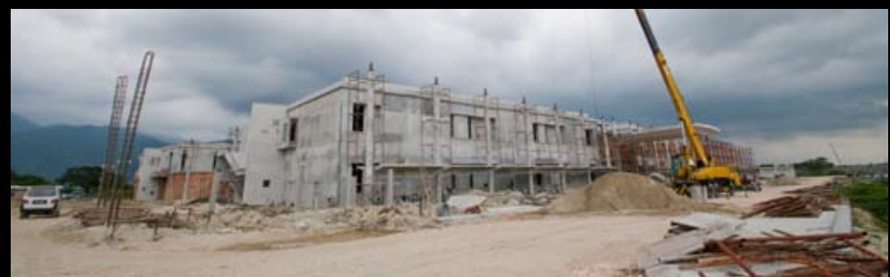
Block N and Block O (under construction) as at 18 November 2011
